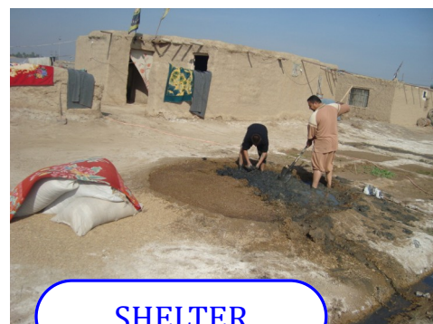
Families in Hay al-Shuhada building a mud house.
